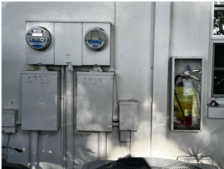
Exterior Master Breaker Boxes
